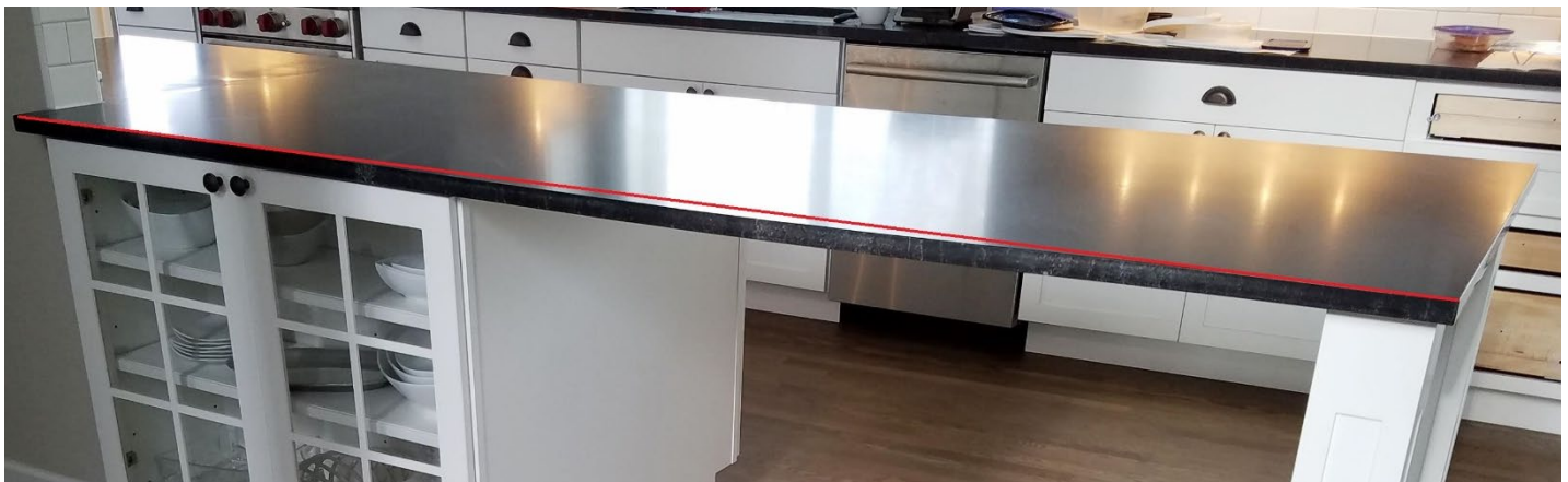
The picture above is an unsupported span of 60". After years without support, the material began to thermoform and sag.
